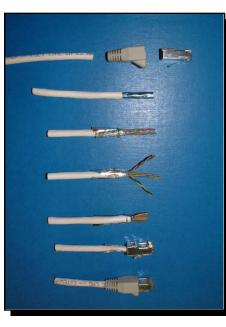
5. Cut Conductors to .500 length to prepare to insert into housing.
